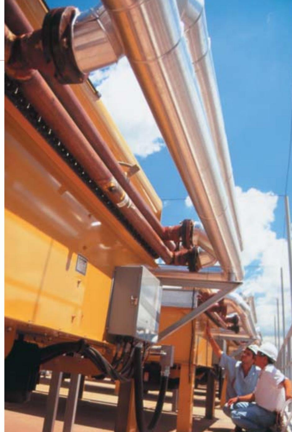
A radiator cools the water that will be used to keep the engine at the right temperature
